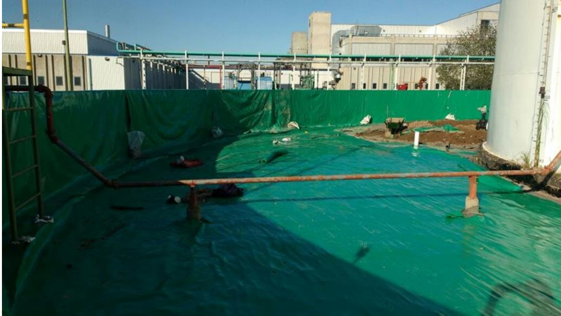
Figure 2: Waterproofing of containment pool with Cipageo Miner
