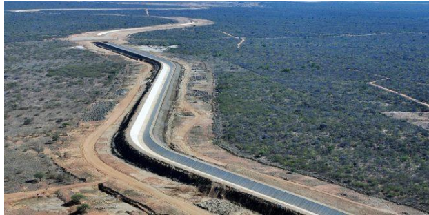
Figure 2: Picture from the construction site
