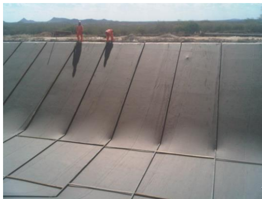
Figure 2: Installation of Cipageo
